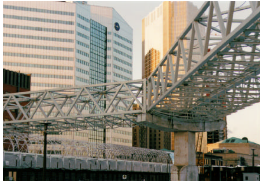
SkyWalk Bridge in its structural skeleton.
