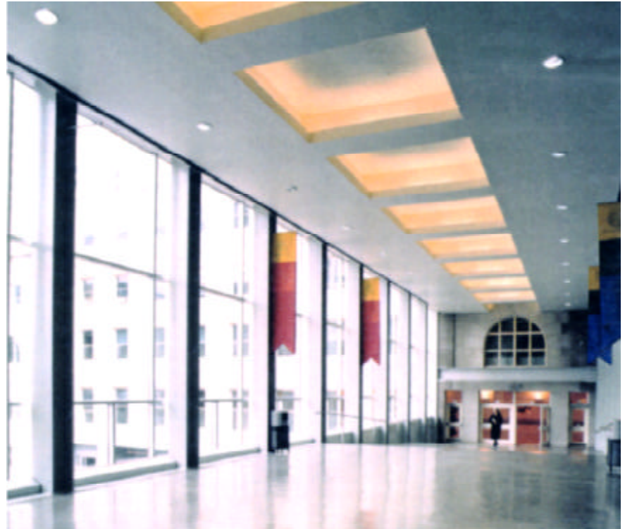
Completed York Street Pedestrian bridge, showing a spacious corridor.
