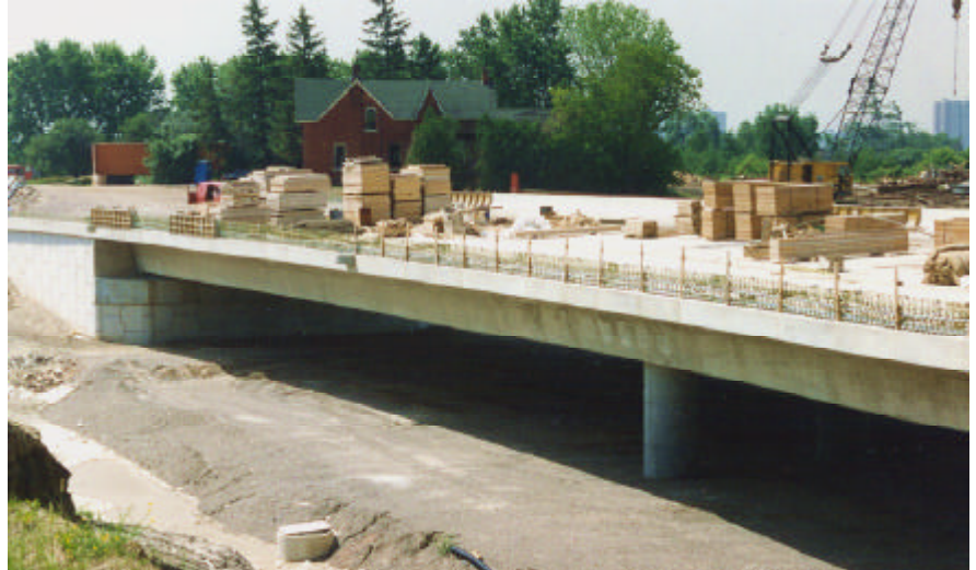
Islington Ave. bridge over Highway 407 deck after post-tensioning.
