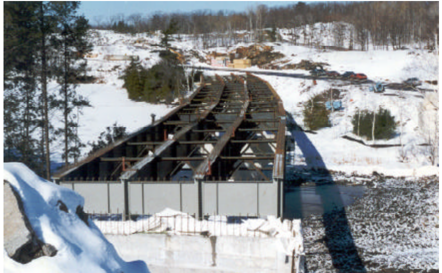
South bound lane structural steel erection completed.
