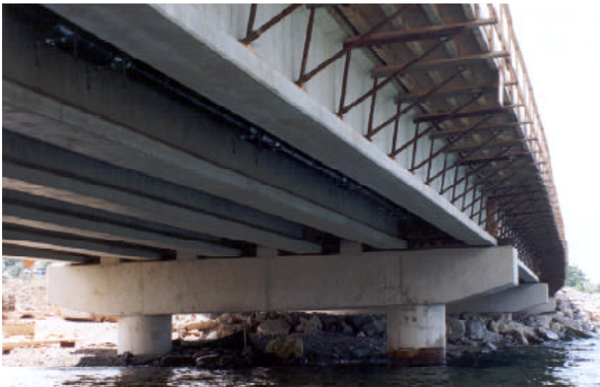
Girder detail at the concrete piers.
