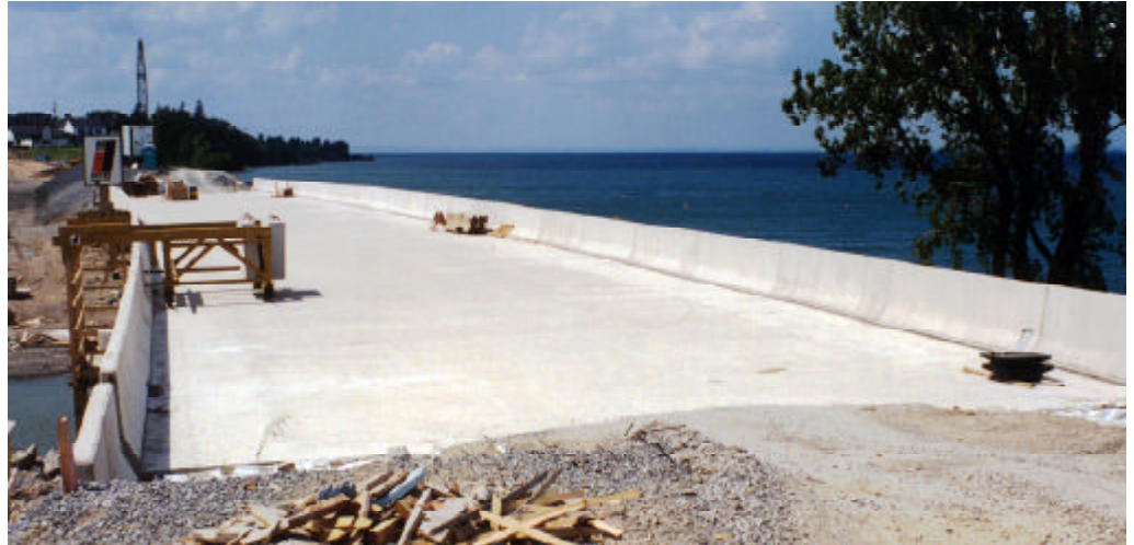
Completed bridge deck.
