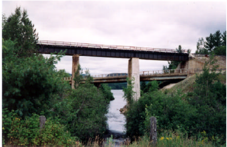
Existing bridge prior to rehabilitation
