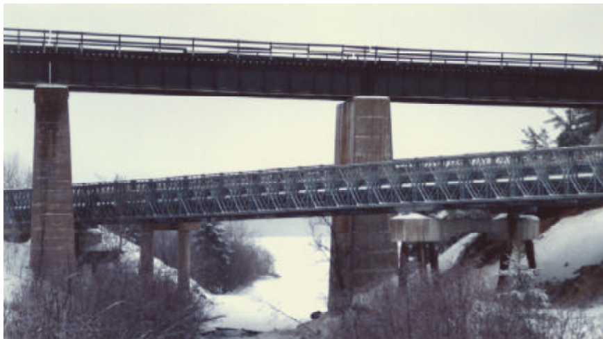
Temporary Acrow structure in place on pile supported concrete pier caps.
