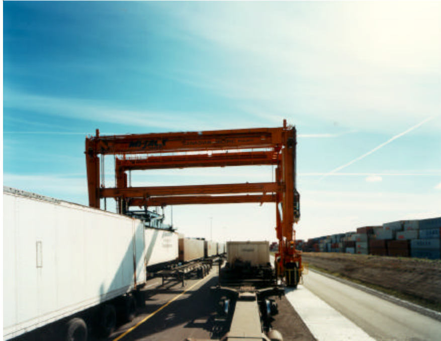
Rubber-tired Gantry on concrete runway double-stacking containers from trailer to rail.
