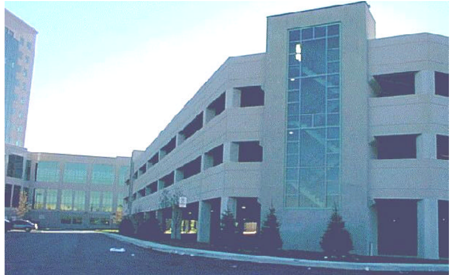
Views of garage showing glazed stairwell details.
