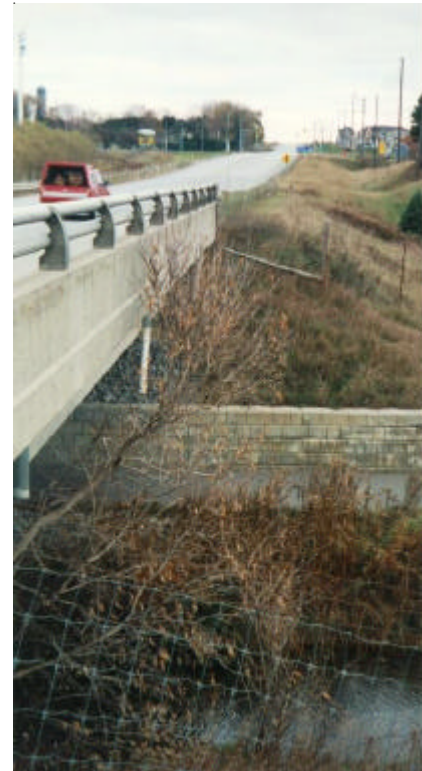
Bridge site at Major Mackenzie Drive over Bruce Creek.
