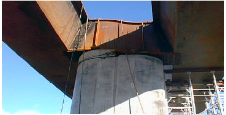
View of integral diaphragm detail at Pier 3
