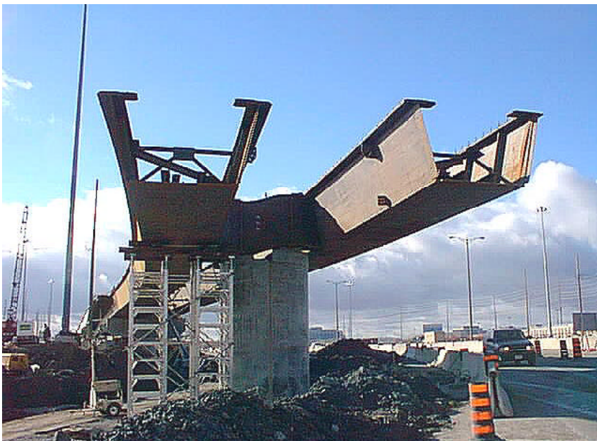
View of girder erection near Pier
