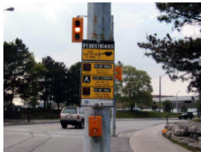
Actuated crossing pedestrian information sign.
