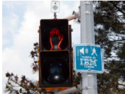
Novax APS Sound Head mounted on pedestrian signal head.
